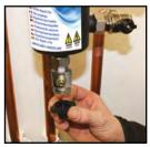
8 Replace cap on drain valve and run the central heating system. Bleed air through air vent if required.
