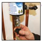
Replace cap on drain valve.
