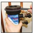
8 Now replace the lid onto the canister and tighten with the Mag Defender spanner. (Do not over tighten).
