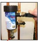
Now the heating system is ready to be filled, ensure the inlet and outlet valves are both in the open position, with the drain valve in the closed position, and then run the central heating system.
