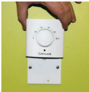
3. After RF pairing is complete on page 7 then slide the thermostat onto the backplate ensuring both sides are engaged. You will feel a positive click when located properly.
